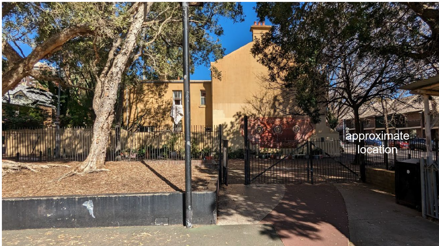
looking south from the basketball courts inside Woolloomooloo Playground
